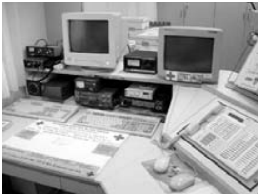
Station in Tulln.
